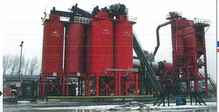
GAZZOLA PAVING LTD. PLANT IN ETOBICOKE, ONTARIO
